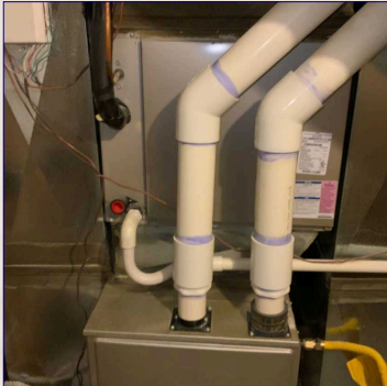
The evaporator coil cabinet
