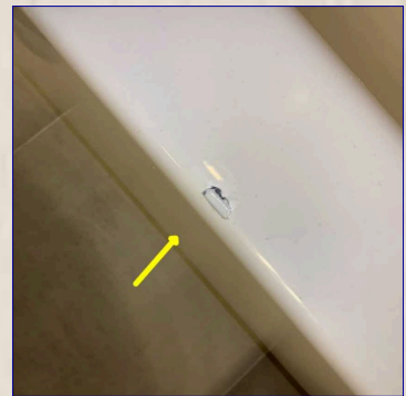
There are chips in the bathtub. Recommend sealing the chips tho help prevent additional damage.
