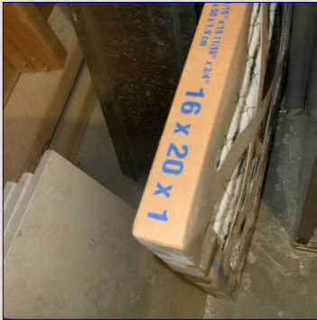
Furnace filter size.
