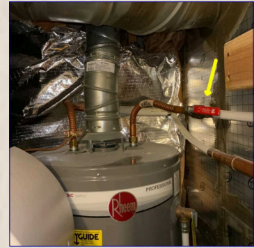
The Water Heater Water Shut Off Valve
