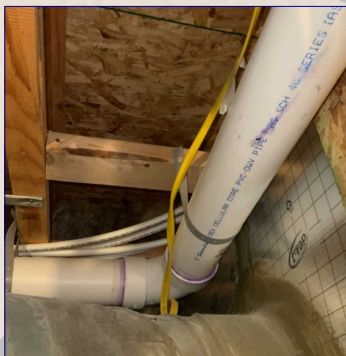
The visible drain/waste piping
