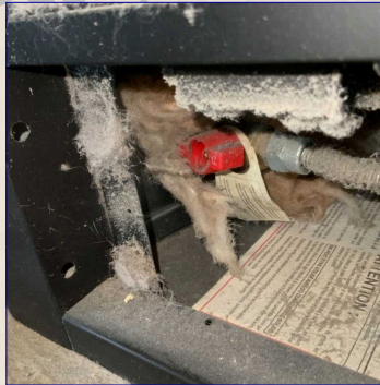
The fireplace gas shut off valve.
