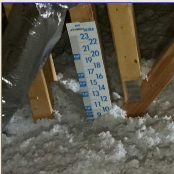
Insulation depth.
