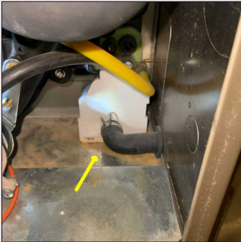
The furnace showed signs of rust and corrosion. Recommend a professional HVAC technician repair or replace as needed.
