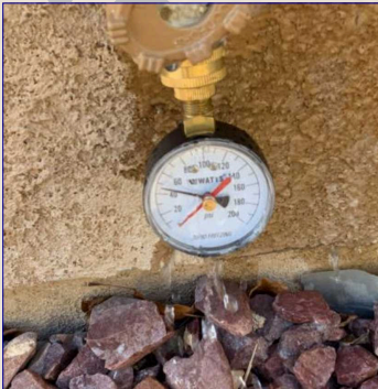
The water pressure at the hose bib.
