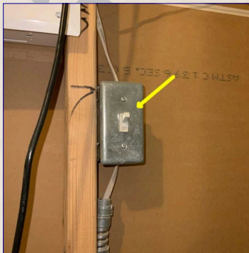
The electrical shutoff switch
